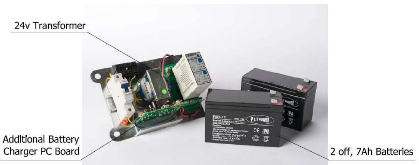
Figure 34: Turnstile control panel with battery backup
